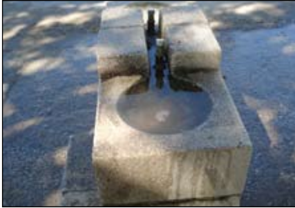
The most common challenge to Drinking Fountains was debris-clogged basins that were unable to drain properly.
