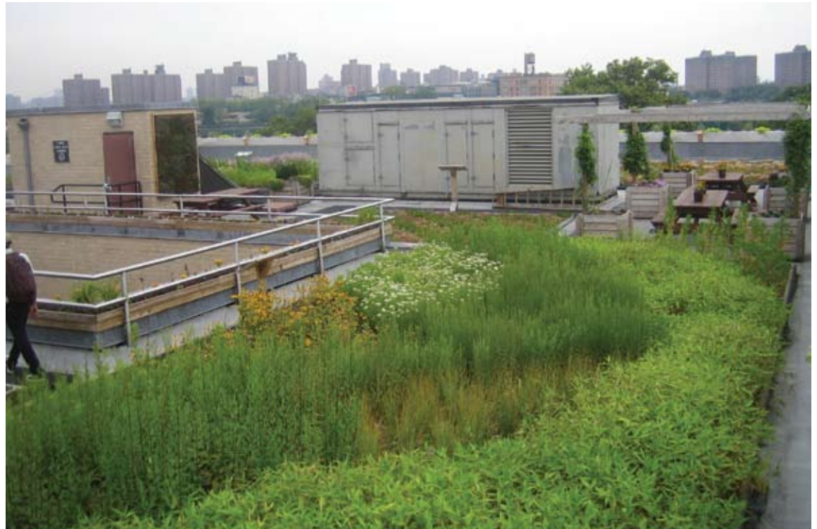
The green roof atop the Department of Parks & Recreation's Five Borough Complex, Randall's Island
